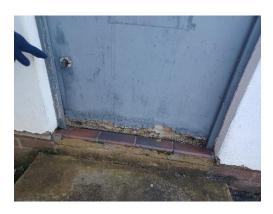
Door located by the commercial bins next to the coffee shop (before the covered walkway). DOCO noted signs of wear (rot) and maintenance required on this doorset. Whilst there was a good lock on the door, it is important to ensure that any maintenance issues are addressed as to not impact the integrity of the door.
